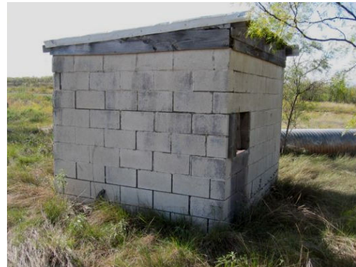
Partially intact low house of skeet field 1
